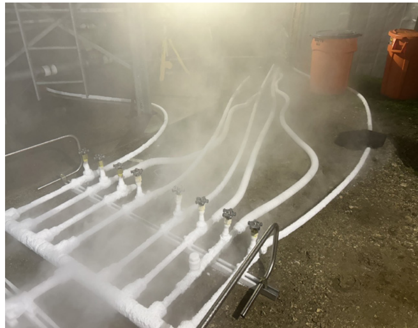
Left: Through pre-established contracts with suppliers, liquid nitrogen is easily sourced and inexpensive. Right: Controlled distribution of nitrogen gas via a manifold and hoses for whole house gassing.
