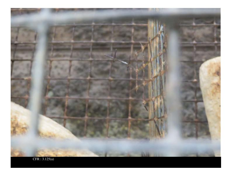
Photographer: SCOTT WELCH Date and Time: Inspection No: 2016082569742232 Description: Close-up of enclosure divider with a loose wire point.
