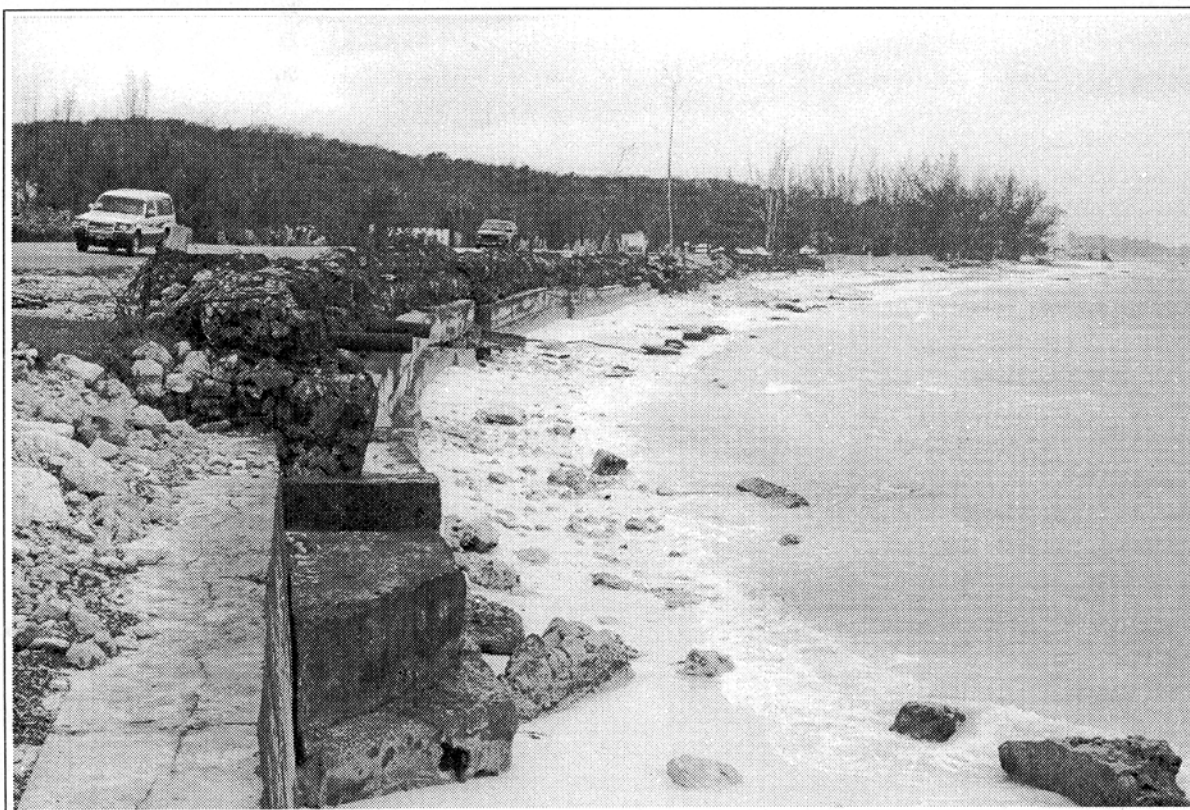
Editorial Figure (see p. 1). A section of the sea wall along the north coast of New Providence about half-a-mile east of Caves Point. In order to protect the road a low concrete wall was built, which encouraged further beach erosion, leading to damage to the wall. The wall has since been heightened several times and is now topped with unstable gabions which are breaking apart. The crude steps in the foreground show the height to which the wall has been raised so far. Both wall and road will be continually eroded unless the road is set back and a broad beach is allowed to develop.
