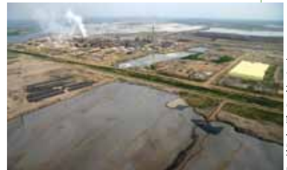
An upgrader plant alongside the open pit tar sands mines north of Fort McMurray, AB; a toxic tailings pond fills the foreground.
